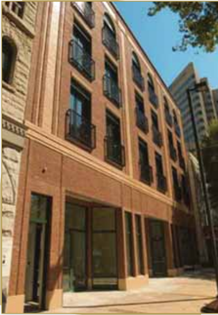
1520 Main Building Exterior
